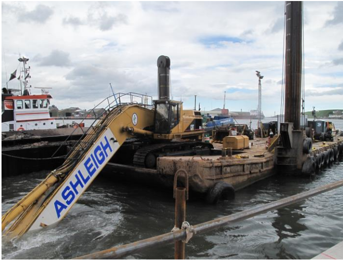
Dredging & Clearance along the new quay wall
