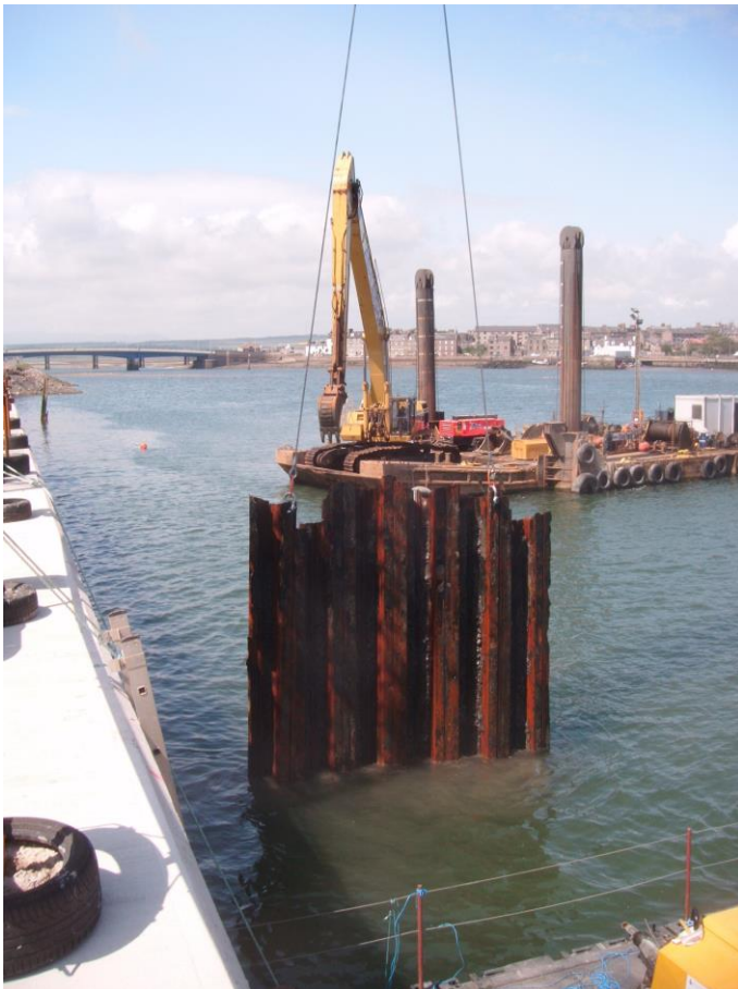
Panel of collapsed sheet piles burned off underwater & being lifted off seabed and set onshore
