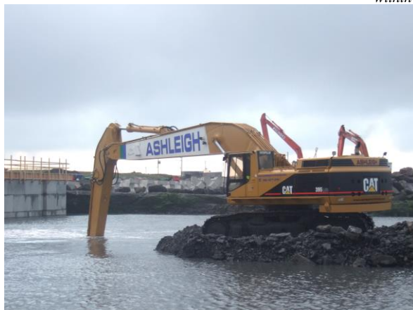
Views of stages of construction including construction of Offshore Breakwater including X Block Armour Units; and dredging of pre-blasted rock within the Harbour Basin
