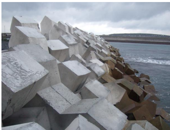
Views of stages of construction including construction of Offshore Breakwater including X Block Armour Units; and dredging of pre-blasted rock within the Harbour Basin
