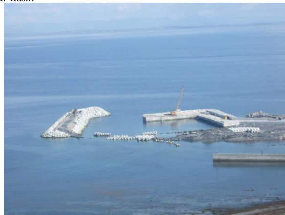
Views of stages of construction including construction of Offshore Breakwater including X Block Armour Units; and dredging of pre-blasted rock within the Harbour Basin
