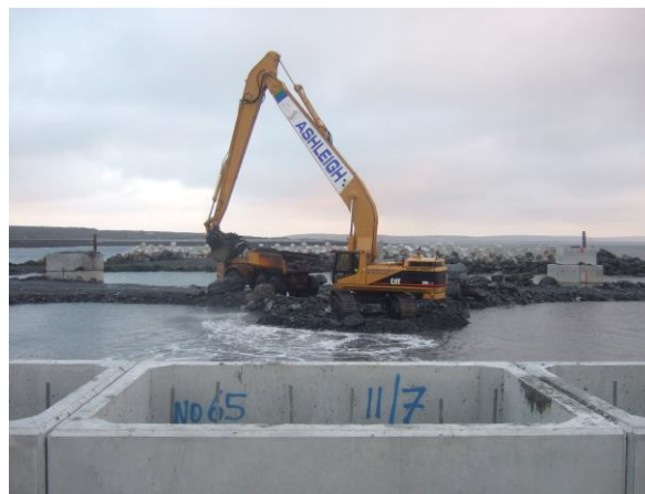
Views of stages of construction including construction of Offshore Breakwater including X Block Armour Units; and dredging of pre-blasted rock within the Harbour Basin
