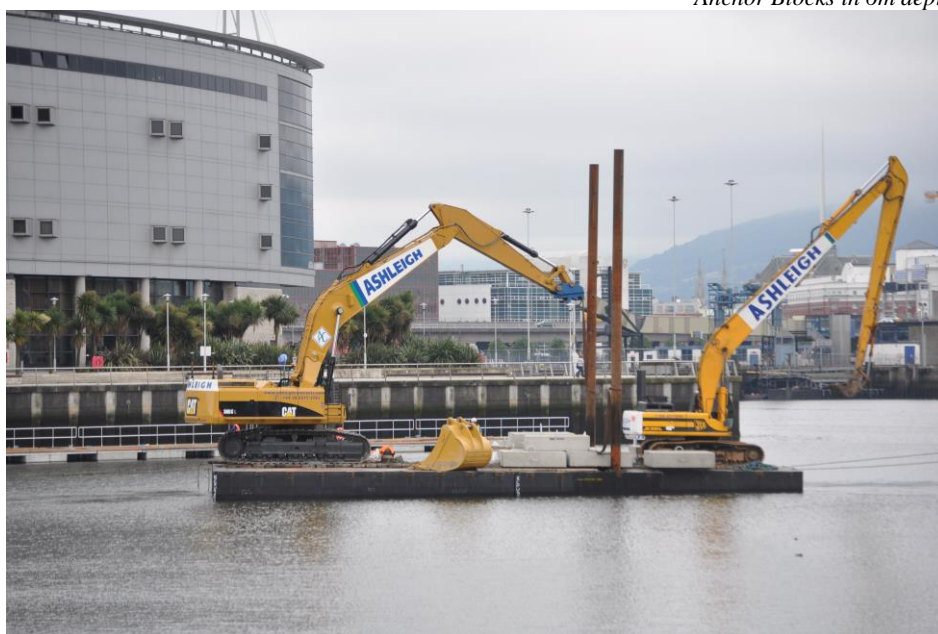
85T Excavator used for placement of 10T PC Anchor Blocks in 6m depth of water
