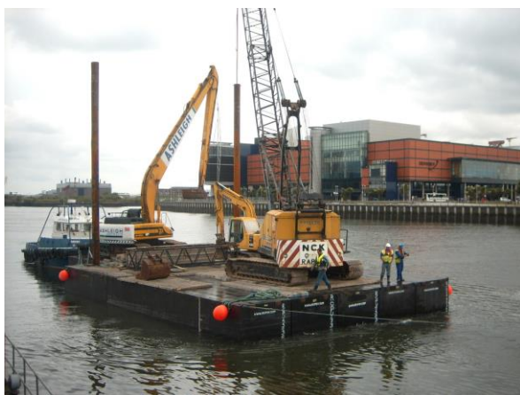
View of Barge with plant for pile driving
