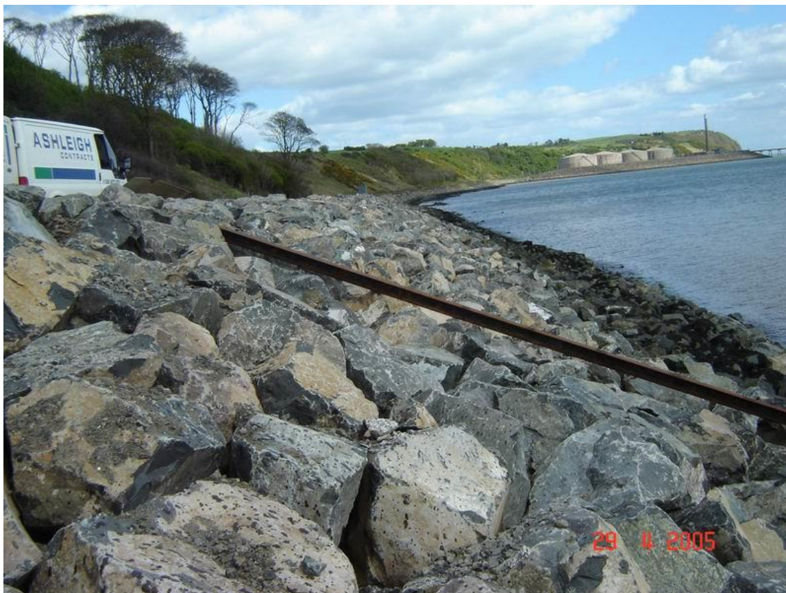
Views of the completed Armoured Revetment at the Saltmins, Kilroot
