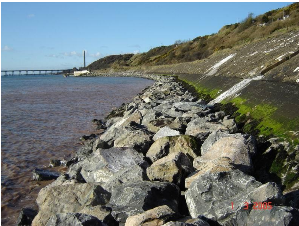
View of the completed Revetment of 3T to 6T Armour
