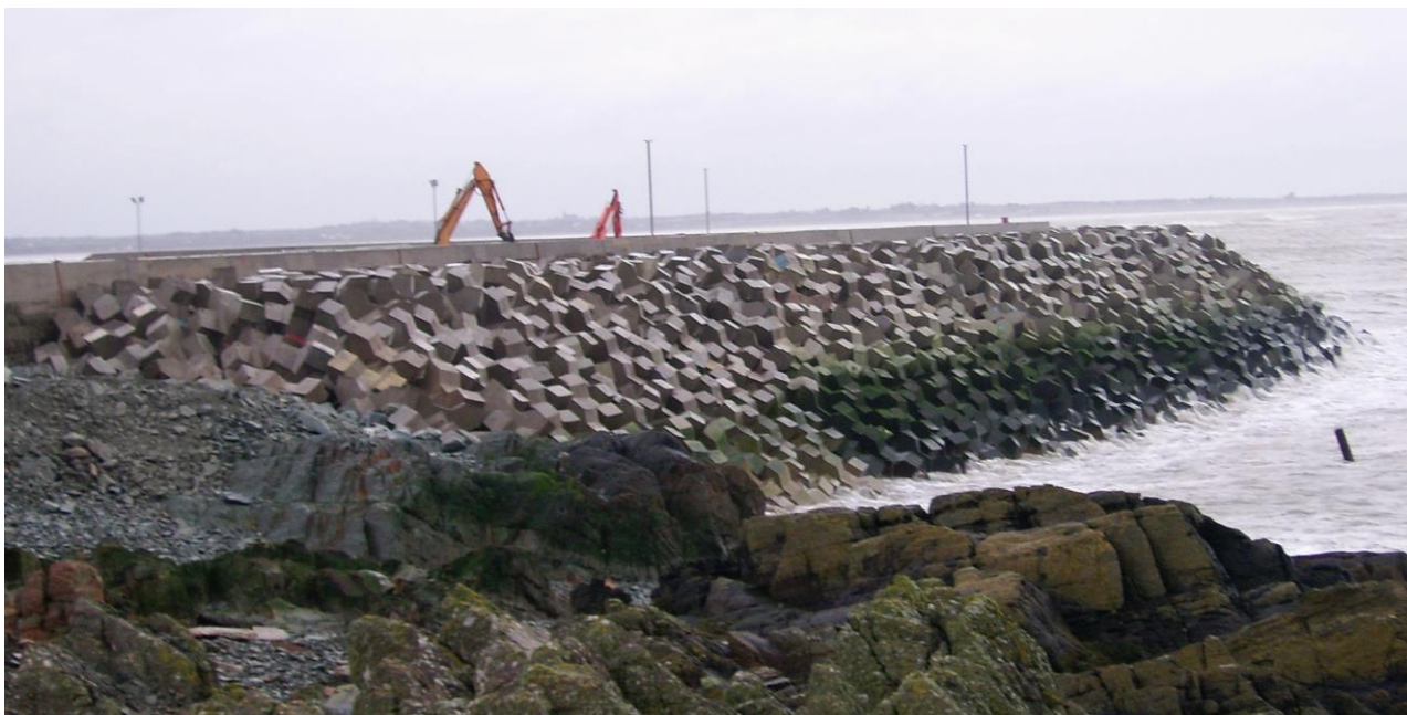
Views showing stages in preparation of rock armoured slopes for and placement of 9.6T Concrete X Block Armouring Units.
