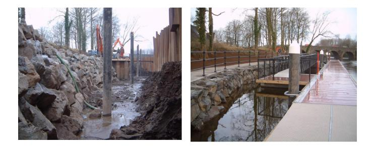
*Views of cofferdam formed to construct rock armoured retaining wall and installation of pontoon piles and the completed works including pontoon installation.*
